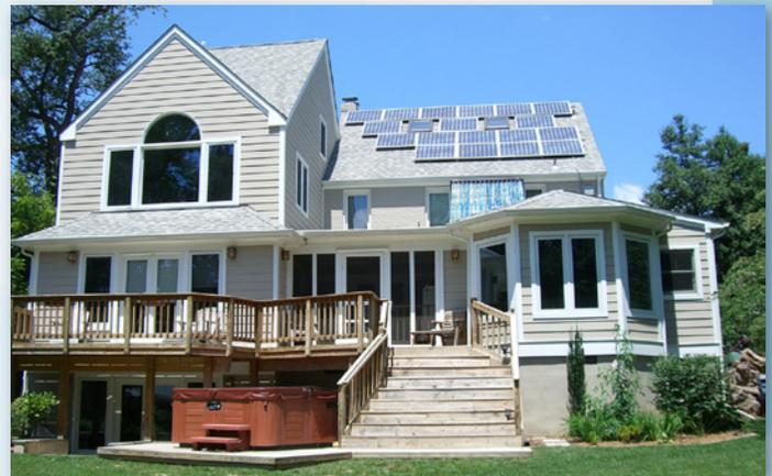
Home in Virginia with 80-gallon evacuated-tube solar water heater and 2.7-kW PV system. *Courtesy: Standard Solar*
