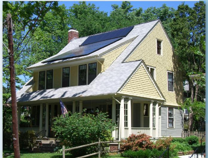
A 6-kW PV system provides 85 percent of this Washington, D.C. home's electricity.
